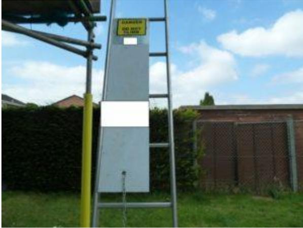
On 6 May 2017, two boys were able to climb the rungs of a ladder within scaffolding erected by Westdale Services at Southville Flats in Cwmbran by placing their feet either side of a ladder guard that did not cover the rungs completely.
